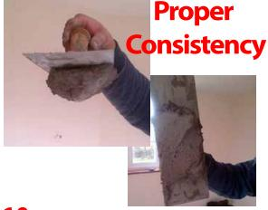
10. The consistency should be such that the material will not drop off the trowel.
