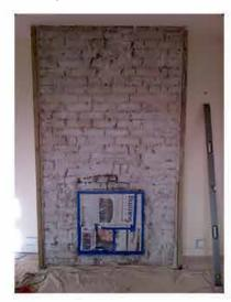
**3.** Attach pieces of wood at each side of the chimney breast at the depth to be rendered.
