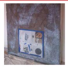
**8.** Coat the render with neat (undiluted PVA) and commence applying the Heat Resistant Plaster when the PVA is tacky.
